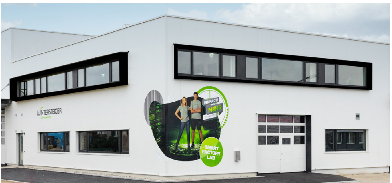
New building 2022: Apprenticeship workshop Smart factory Lab and Technik & Service Seedmech
